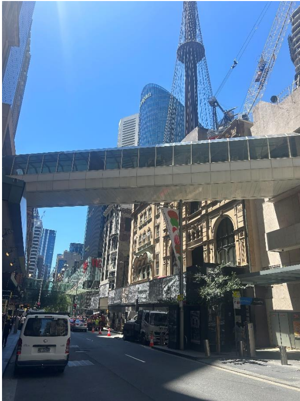
Figure 7 Sky Bridges – Pitt Street (left) and Castlereagh Street (right)
